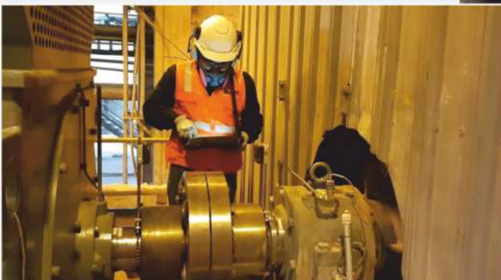
Cooling Tower Fan Alignment
